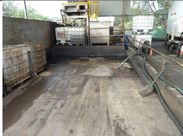
Photo 3: Truck discharge bay and bund
