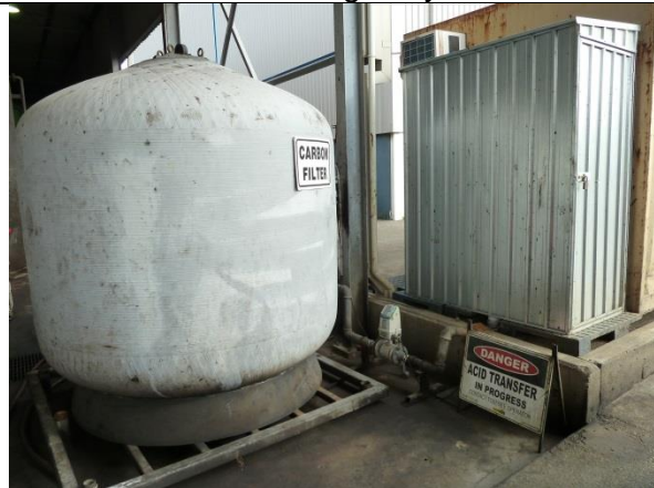
Photo 5: Carbon Filter and Sample Shed (sewer discharge point within)
