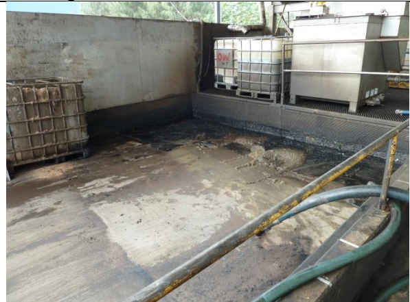
Photo 4: Truck discharge bund
