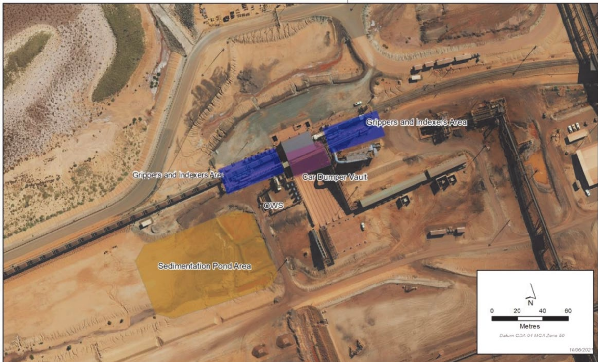
Figure 1: Car dumper and proposed sedimentation pond area
